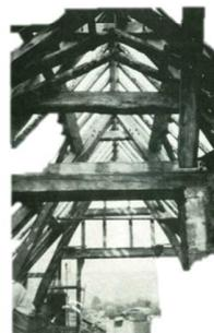
Assembly of roof support structure; raising up of the timbers into position and interior view of completed roof support.
